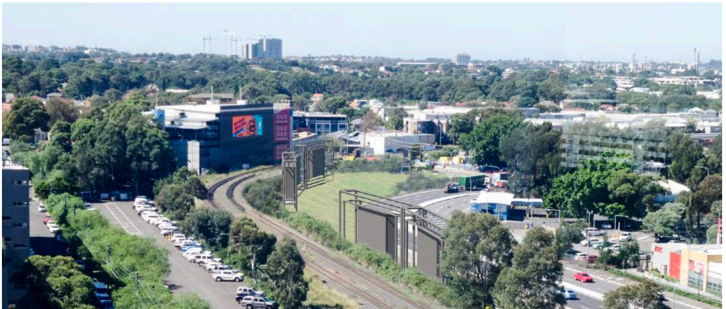
Above: Photomontage illustrating the duplicated Botany Line, looking southeast towards Port Botany
