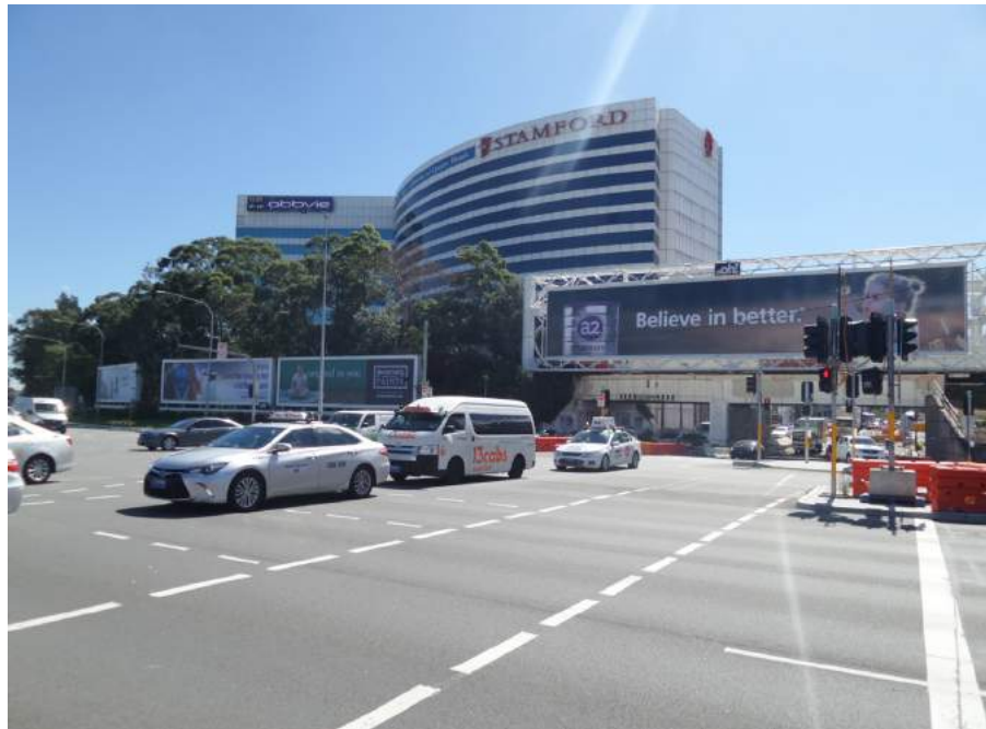
Above: Existing rail bridge over O'Riordan Street, Mascot
