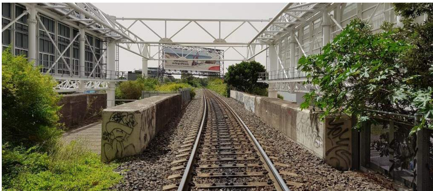
Above: Image of existing Botany Line at O'Riordan Street, Mascot
