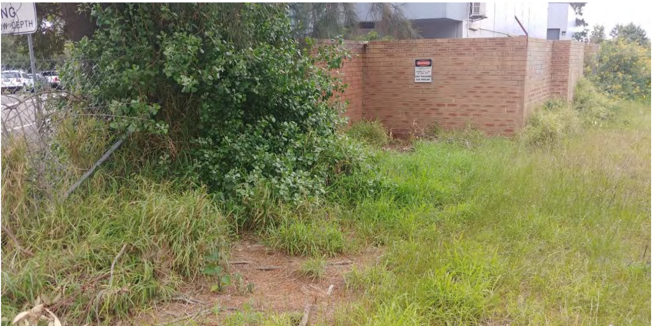
Figure 6-2 Signage within rail corridor indicating high pressure pipeline
