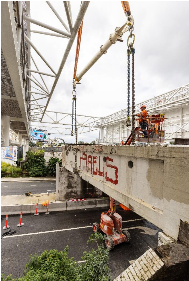
Removal of a 62-tonne bridge girder on O’Riordan Street bridge
