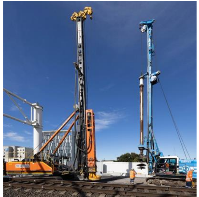
Piling work commences at the O’Riordan Street bridge
