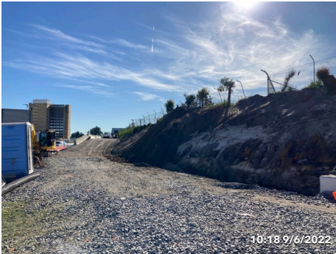
Photo 10 Retaining walls along Qantas Drive
