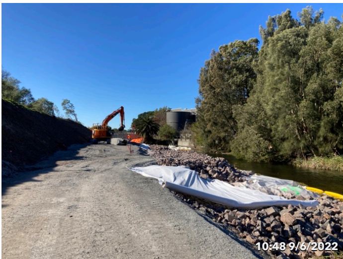
Photo 30 Piling pad preparation
