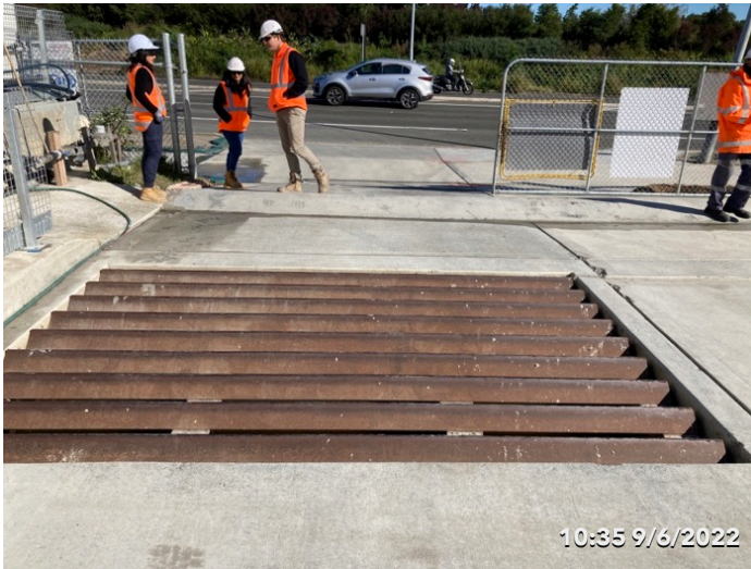
Photo 19 Rumble Grid at Botany Triangle
