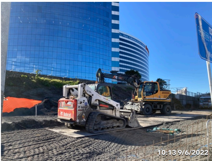
Photo 6 Stamford Hotel - Cleared area - Piling pad
