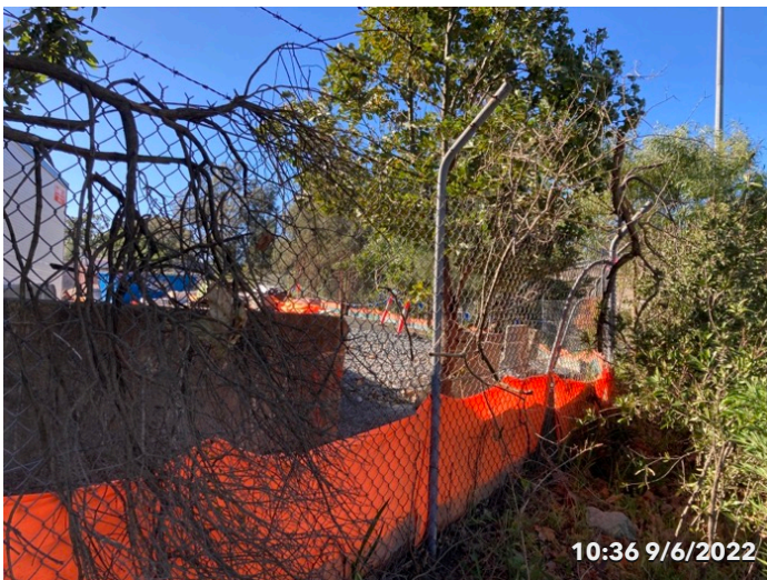
Photo 21 Mill Pond Compound - silt fence installed around the perimeter
