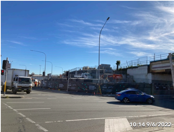
Photo 7 Retaining wall and embankment was built with Gateway Project
