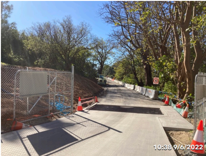
Photo 22 Mill Street Access track stabilised paved access with rumble grid
