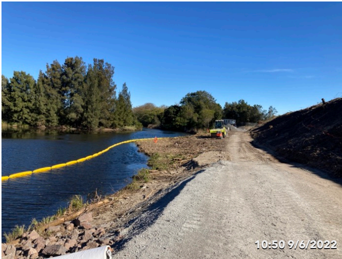
Photo 31 Road improvement area at Mill Street. Silt curtain was installed.
