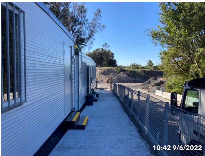
Photo 27 Site Shed at Mill Pond
