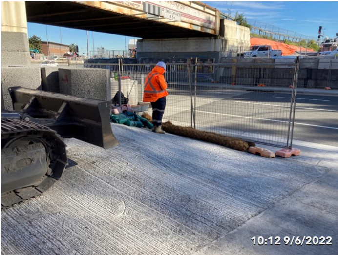
Photo 4 Sediment controls installed at Robey St access/egress
