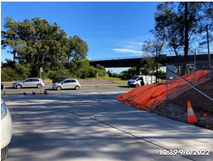
Photo 23 Botany Road - neat access/egress
