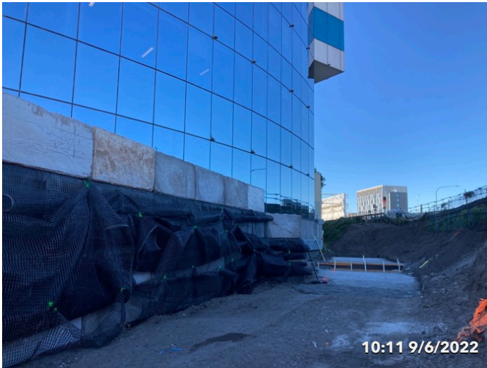
Photo 1 Retaining wall adjacent to Stamford Hotel
