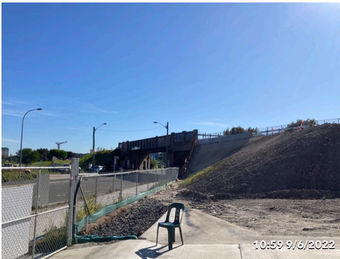
Photo 35 Heritage listed bridge
