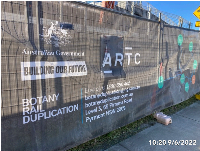
Photo 13 Shade Cloth around the work perimeter
