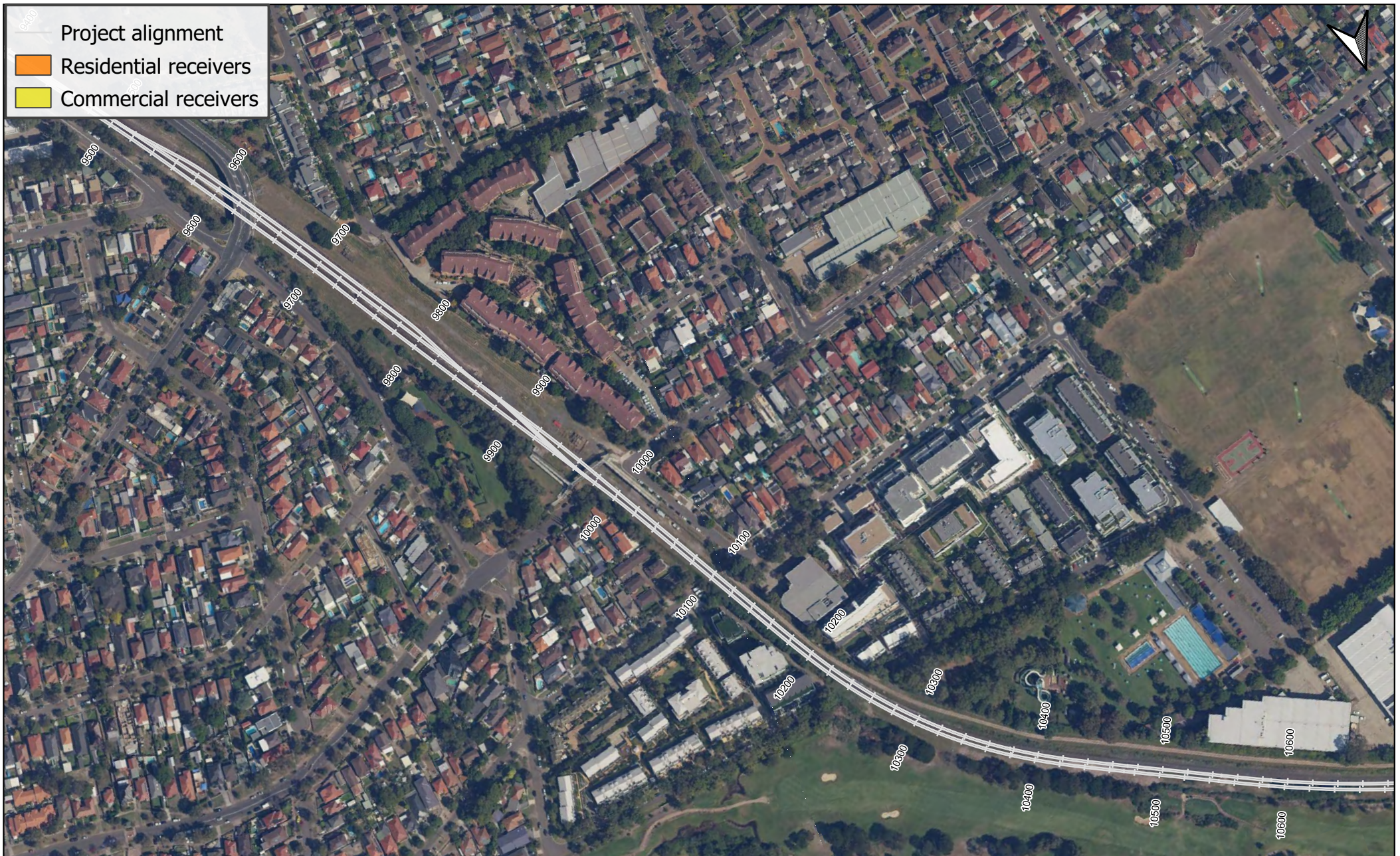
Year 2034 Build Scenario - With EPA Licencing and Lubrication Sensitive Receivers Exceeding Noise Criteria
