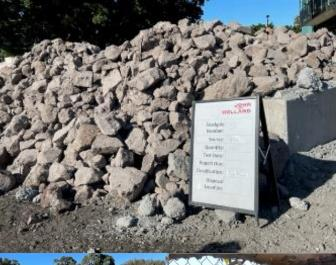
Stockpiles labelled appropriately. Survey picked up of the floor is 7.5RL Top of pile is 9.9RL. The height of the stockpile is approx. 2.4m and compliant
