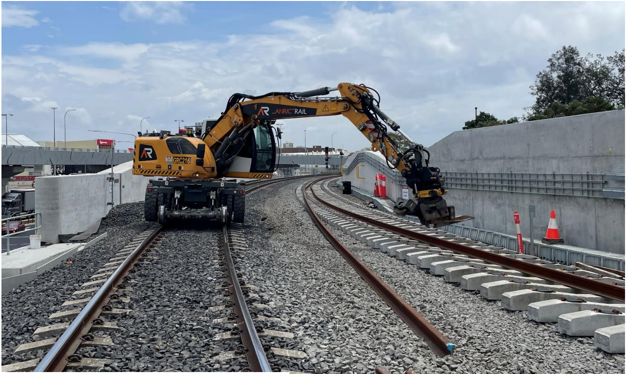
Installing new rail track at Robey Street bridge
