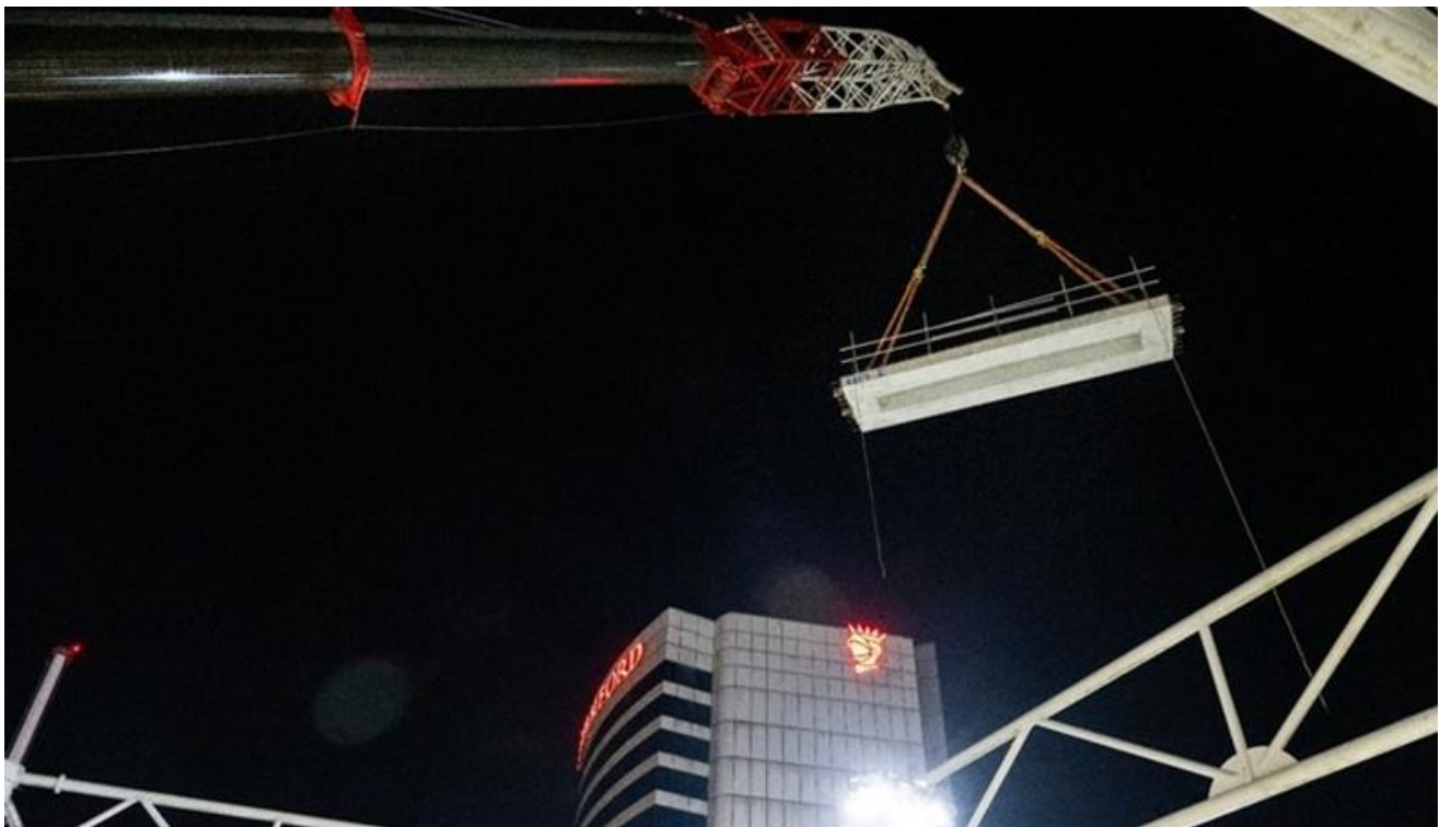
Crane lifting in new bridge planks at O’Riordan Street bridge during the shutdown
