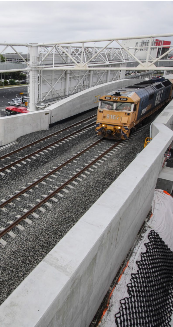
The first train uses the newly-commissioned track over O’Riordan Street bridge at Mascot
