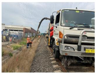
There are only a few times a year we can access the rail corridor safely to do major works. Over a weekend in January 2022, we were able to get plenty of work done including signalling works and design investigations, as well as excavations for new cabling.
