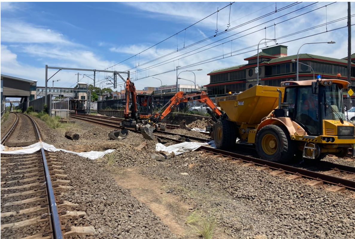
Below – Triple Track underground crossing construction at Cabramatta Station during weekend possession WE31
