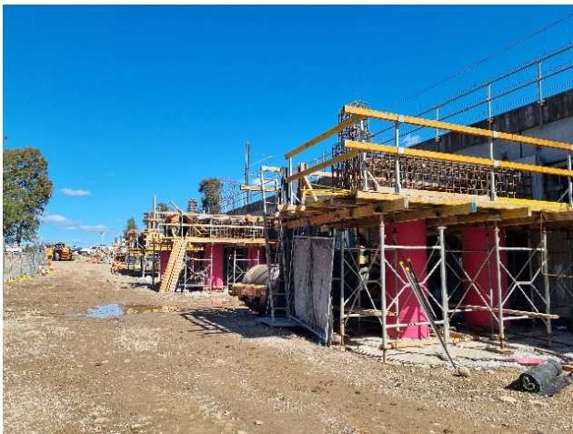
Cabramatta Creek bridge form work
