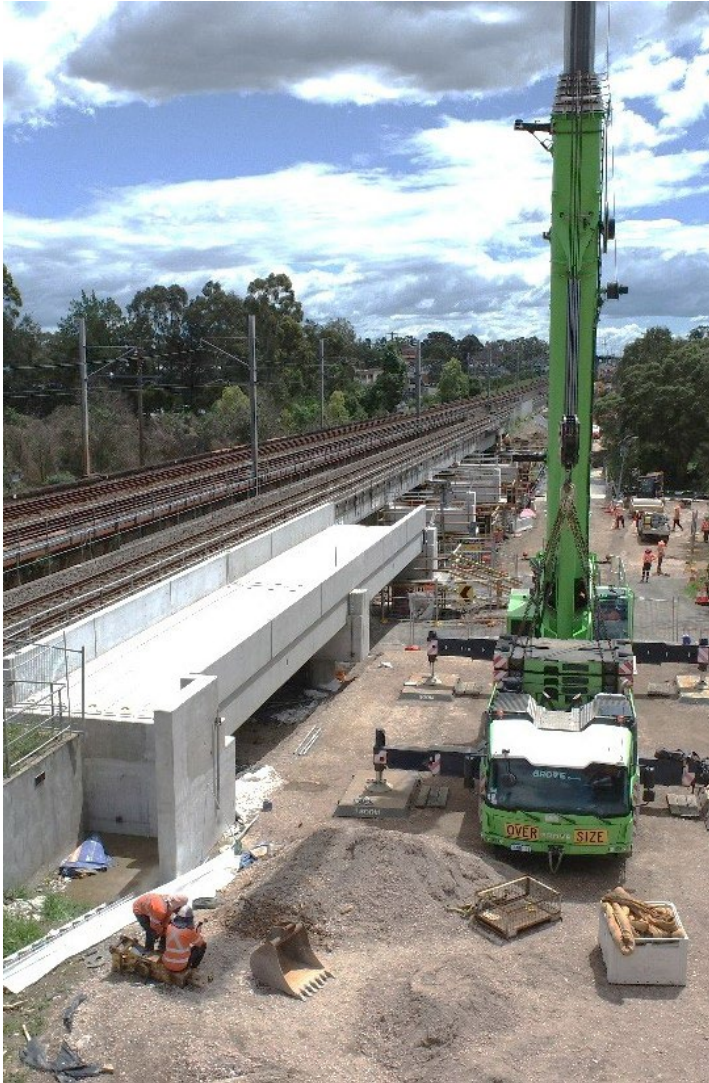
The new rail bridge at Cabramatta Creek is taking shape.
