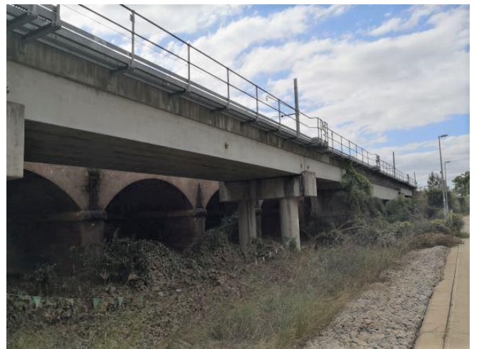
The existing rail bridge at Cabramatta Creek
