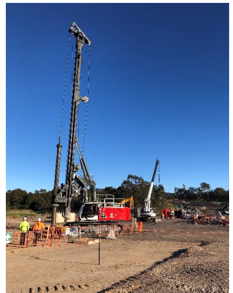
Example of a piling rig used for the bridge foundation work
