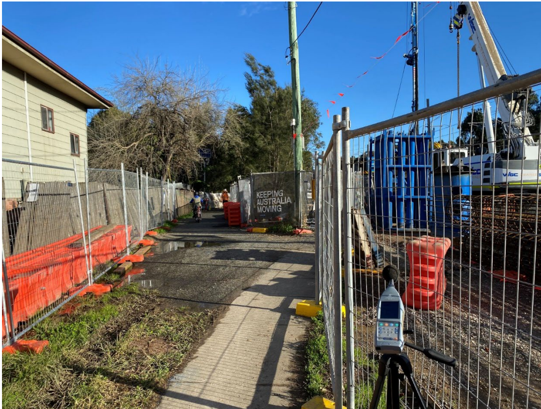
Above: Spot check at 10 Sussex St during piling activities in July
