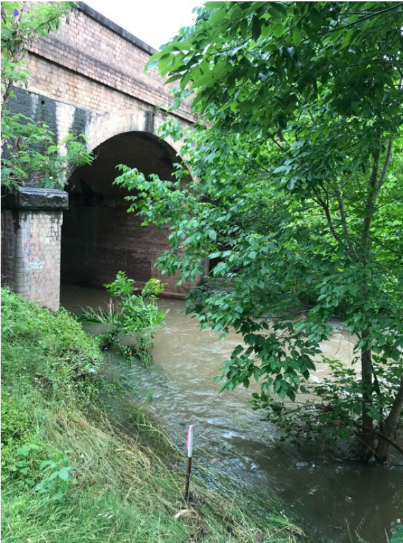
Above: Upstream Surface Water Sampling Point SW1 Latitude: -33.90260 ° Longitude: 150.93804 November 2021
