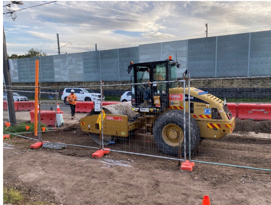
Above: Monitoring at 170 Broomfield St on July 12 th 2022 during compaction rolling.
