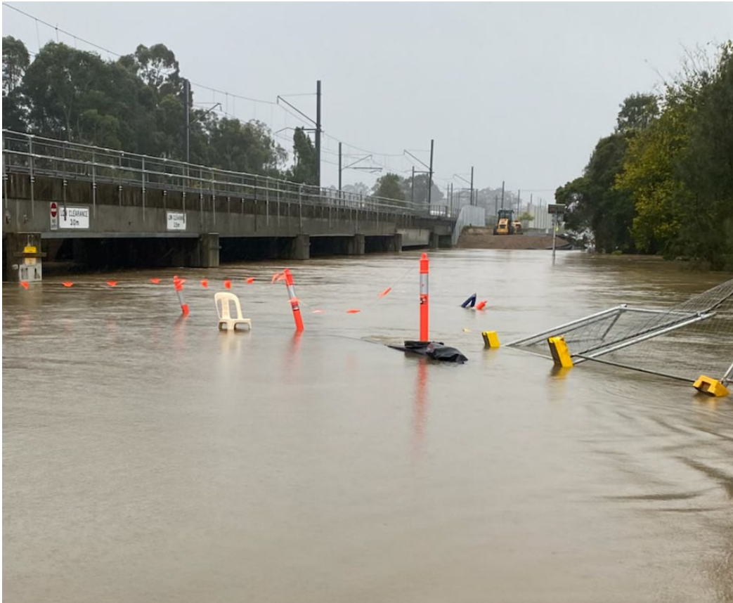
Above: July Floods at Cabramatta Rail Loop 2022
