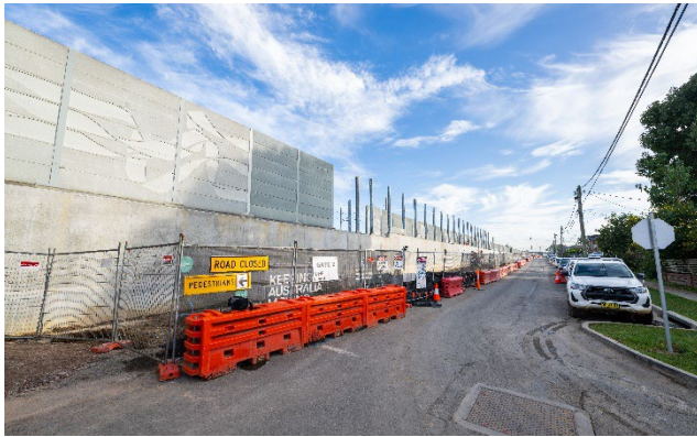
Noise wall works in Broomfield Street.
