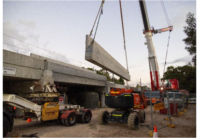
A plank being installed on the new Cabramatta Creek bridge.
