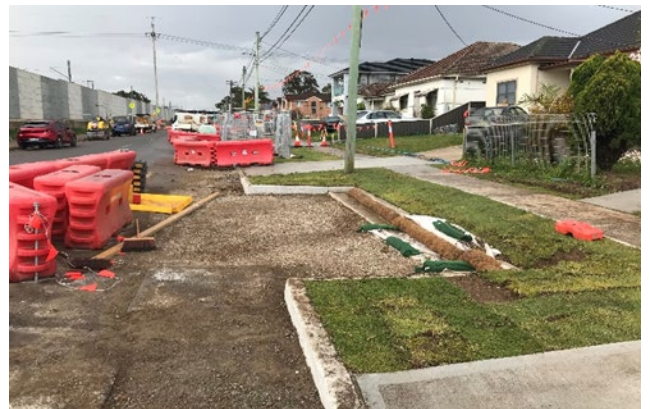
Road works on Broomfield Street.
