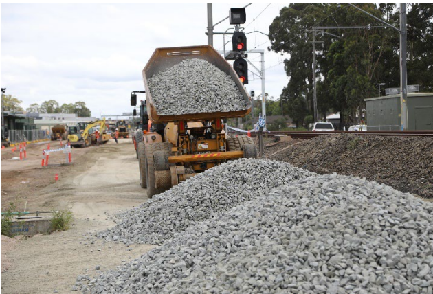
Work underway as part of the track realignment
