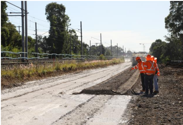
Engineers inspecting the foundation where the new track will be laid
