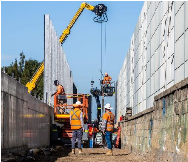
Relocating existing panels onto the new retaining wall
