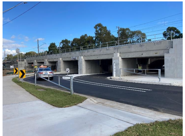
New Sussex Street bridge
