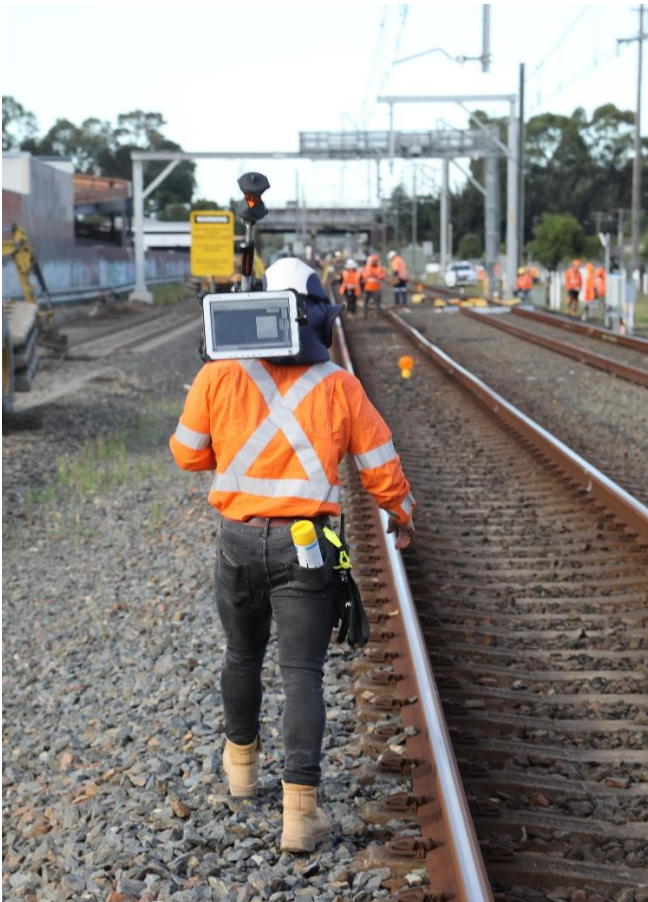
Surveyor marking survey points along the track during the rail shutdown.
