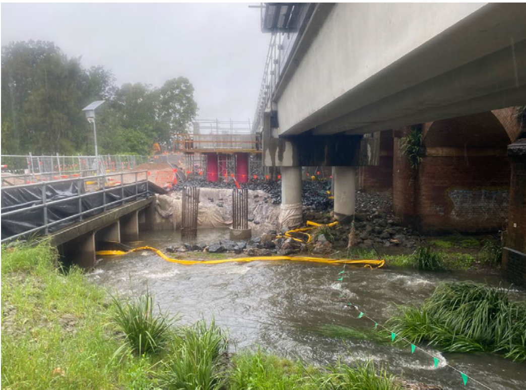
Above: Upstream Cabramatta Creek during a minor rainfall event in November 2022
