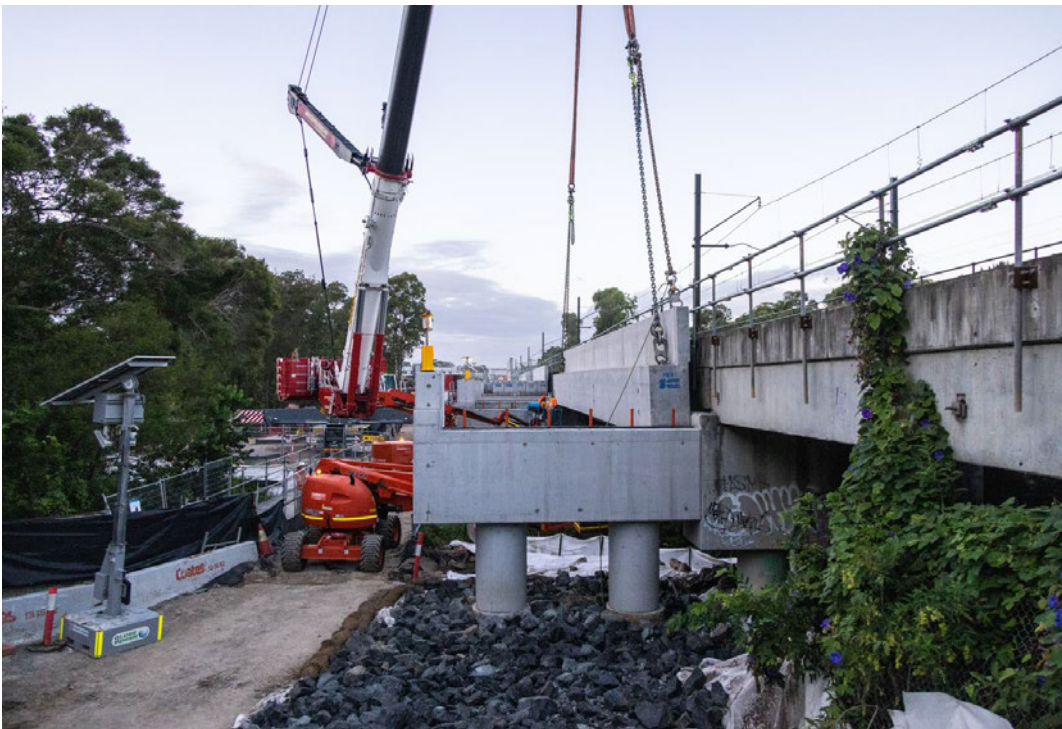
Above: Progression of bridge works at Cabramatta Creek during March 2023.
