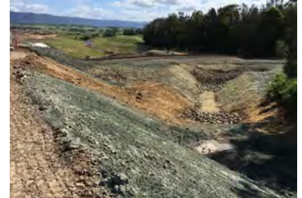
Figure 8 - progressive and early stabilisation as works progress
