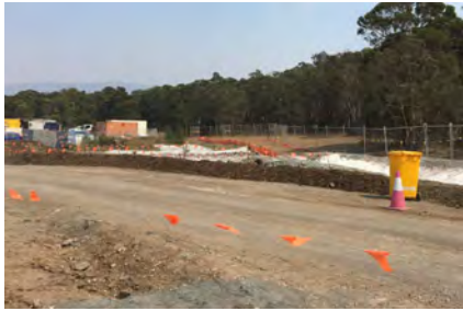
Figure 4 - mulch filter bund installed adjacent to a waterway
