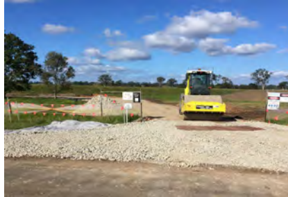
Figure 6 - construction access and egress with a vibration grid
