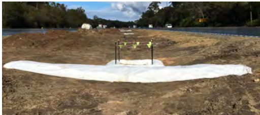
Figure 5 - pit protection with downslope earth bund
