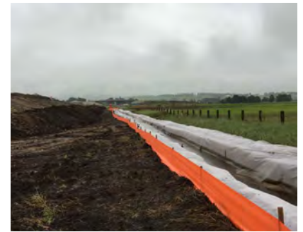
Figure 9 - sediment fence installed alongside a clean water drain
