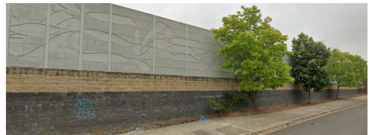
Existing Retaining Wall
