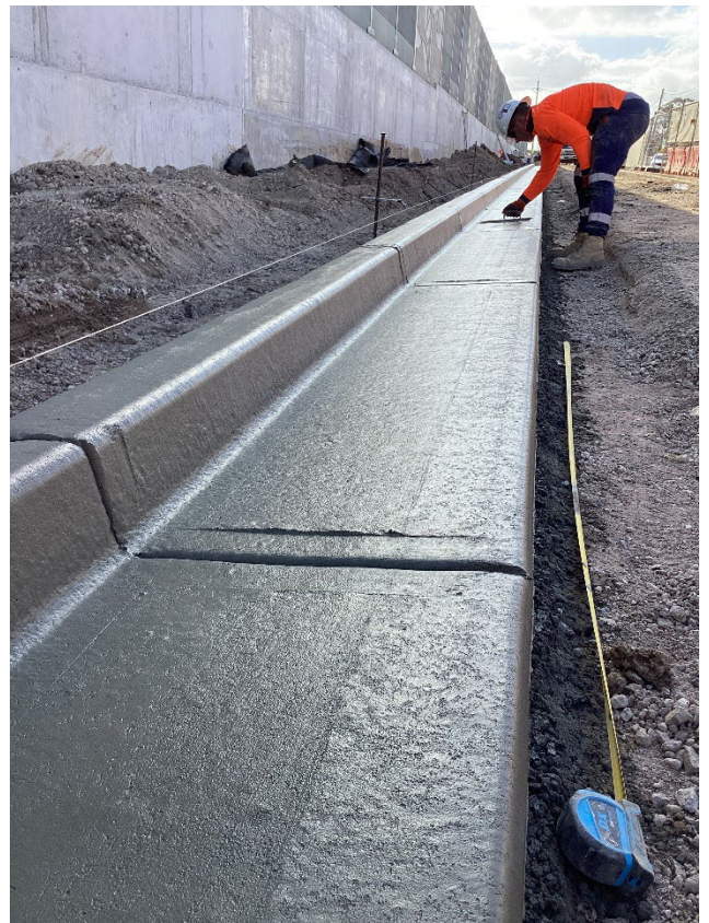
Completing the Broomfield Street western kerb
