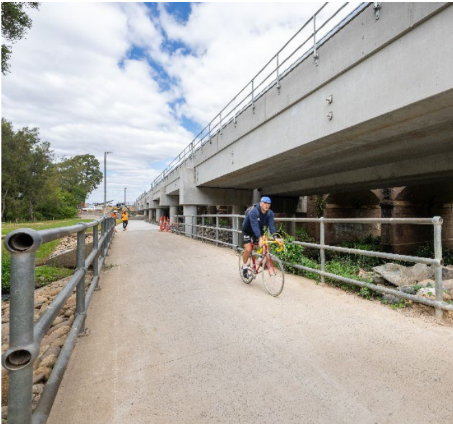
New shared path adjacent to Cabramatta Creek Bridge
