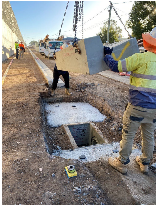
Installing a concrete kerb over the newly built drainage network
