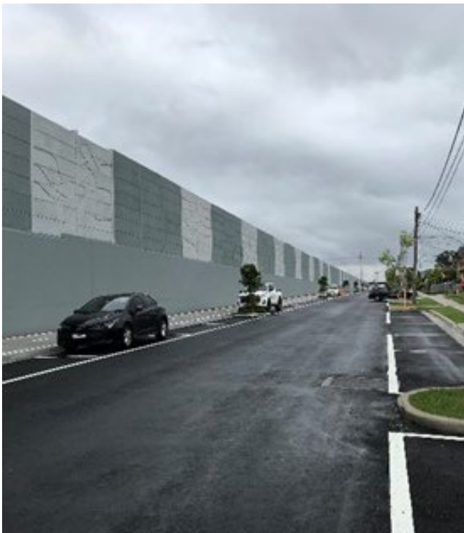
Newly painted noise wall, asphalt and line marking along Broomfield Street
