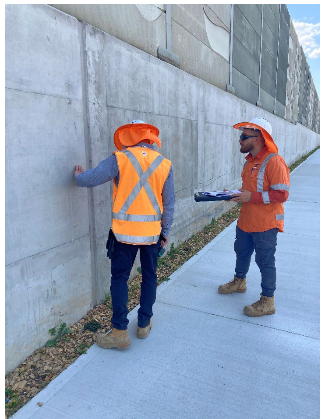
Engineers inspecting the new retaining wall on Broomfield Street
