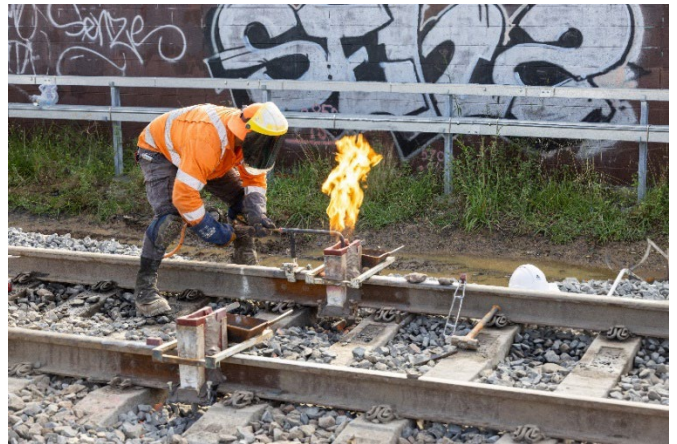
Rail track welding activities
