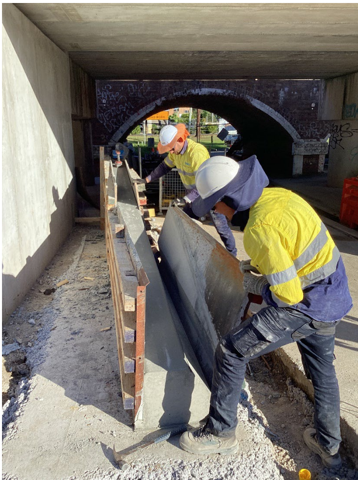
Construction of concrete traffic barrier at Sussex Street Bridge
