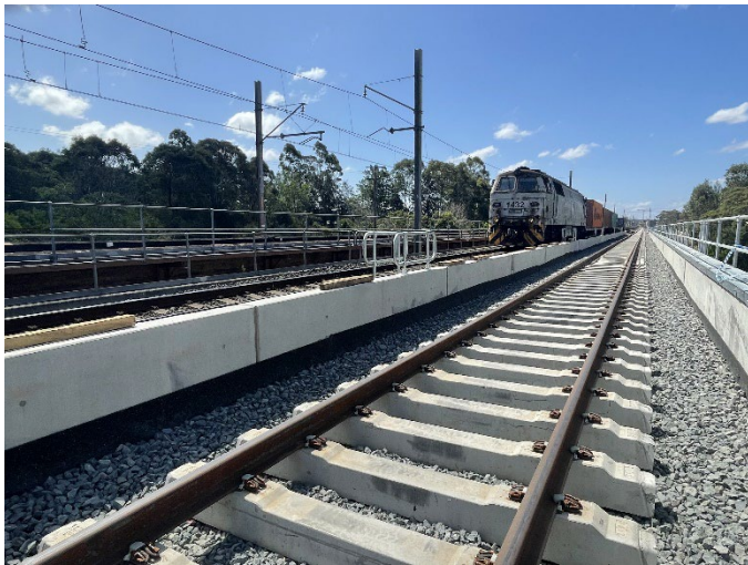
Newly laid track on the Cabramatta Creek Bridge
