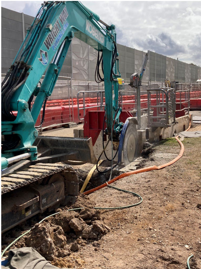
Road saw cutting the area for the new drainage pipe
