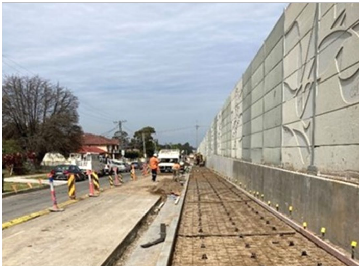
Building the new share path along Broomfield Street
