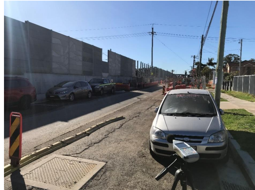
Above: Monitoring at 150 Broomfield St (NML2) during July 2023.
